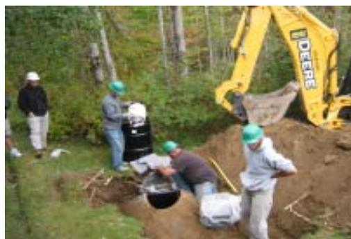
Cleaning an underground storage tank at Silver Towers before removal.
