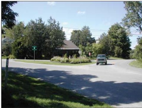
lines, especially for cars exiting the bridge. Redesign of the triangle would help improve pedestrian safety and vehicle circulation. One option would be to remove the triangle and T the intersection, bringing all traffic to a 3-way stop. This would provide excellent sight lines and significantly improve pedestrian and vehicular safety. By removing asphalt, more green space and vegetation could also be introduced and more efficient pedestrian walkways and amenities would result such as
