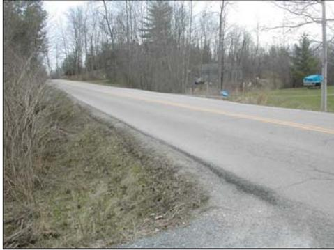
Currently, the roads in the study area do not have continuous white edge stripes (fog lines) to distinguish shoulders from the travel lanes, as seen in the picture below. The need for road markings of all types is becoming increasingly important in controlling the position of moving traffic into orderly lanes and in showing the road user where he can and cannot be on the roadway. Striping helps moderate vehicle
